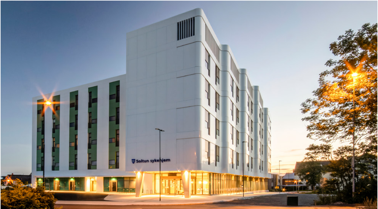
Sola Sykehjem Hospital | Sola, Norway | STB - S10
